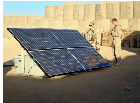
Two Man Transportable Solar Power Sources Deployed for Power at a Remote USMC Patrol Base in Afghanistan
