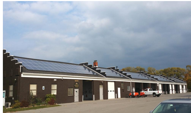
Pitched Roof Solar Power Systems
